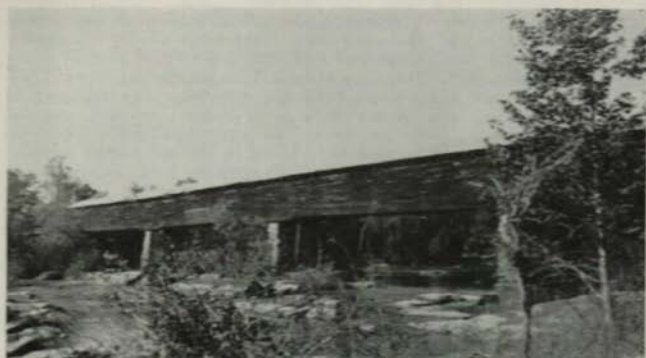
The covered bridge on Alabama State Highway 49, near the Historic Horseshoe Bend Battleground, was erected in 1908. It is held together largely by wooden pegs. It is about 12 miles north of Dadeville.
