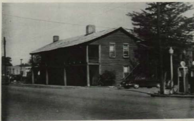
This building was originally the United States Hotel, and was erected about 1836. It has been owned by the Dennis family for more than a century and has been known as the Dennis Hotel most of that time. It was in this hotel that Johnson Jones Hooper wrote many of his humorous stories, among which were the ADVENTURES OF SIMON SUGGS. This building is located at Dadeville.
