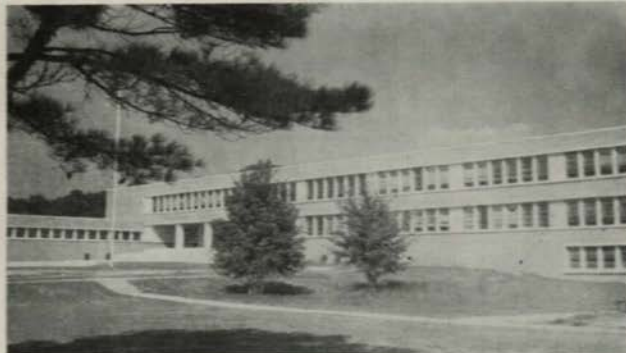
A view of the half million dollar Benjamin C. Russell High School at Alexander City. Erected since World War II, this building embodies the very latest features in educational plants.
