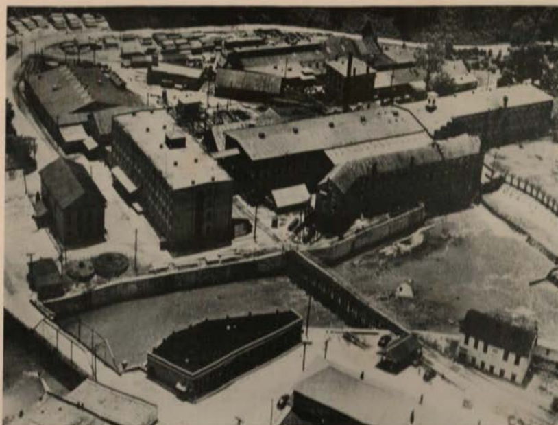
CONTINENTAL GIN COMPANY PLANT on Autauga Creek at Prattville, Alabama.
