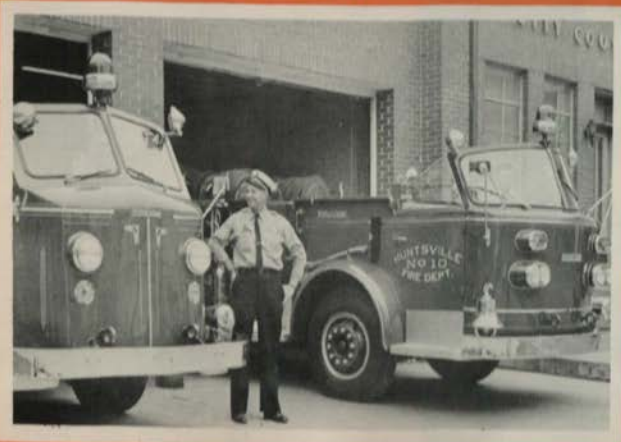
Fire Chief Tolen checks new equipment.
