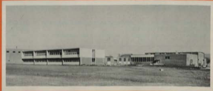
The Westlawn School, where new gym, auditorium and lunchroom were added at a cost of $487,000.
