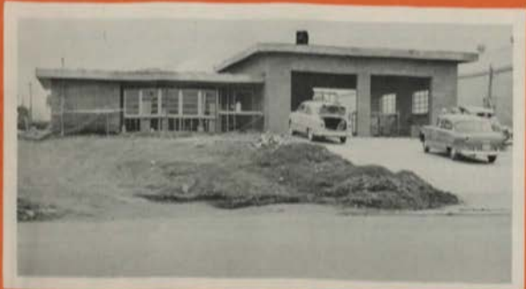
Nearly completed fire station on Highway 72.
