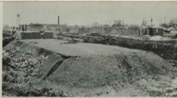
Construction starts on a new low-rent housing project.
