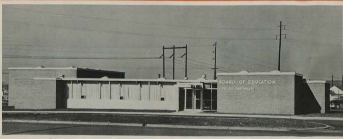
The modern building in which the board of education is housed.
