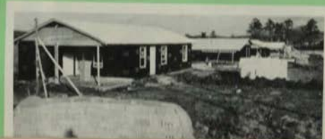
A typical subdivision under construction.
