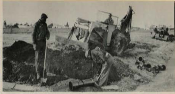
Gas main installation.
