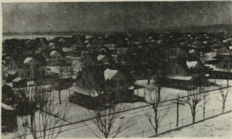
This bird's-eye view illustrates the monotony of mill architecture. These rows of identical duplexes are from the Merrimack village.
