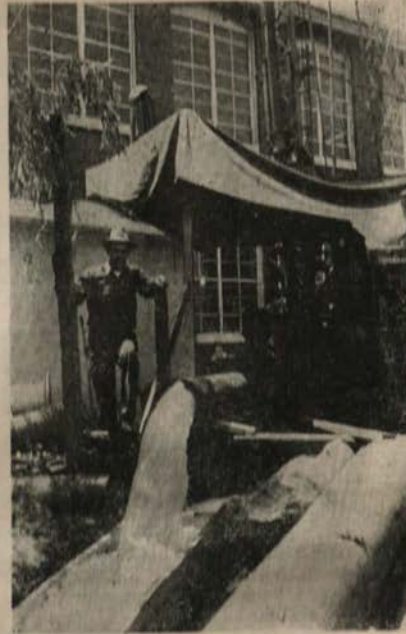
Plate 23-B.—Pumping test on well Q-79 at General Shoe Corp. at approximately 1,000 gallons per minute.
