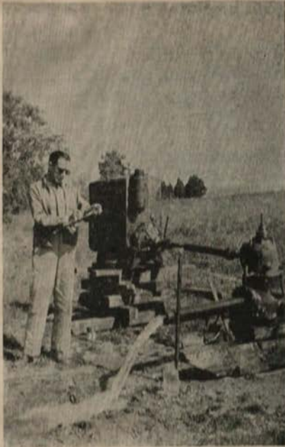
Plate 23-A.—Typical installation used in pumping tests on test wells. Well pumping approximately 100 gallons per minute.
