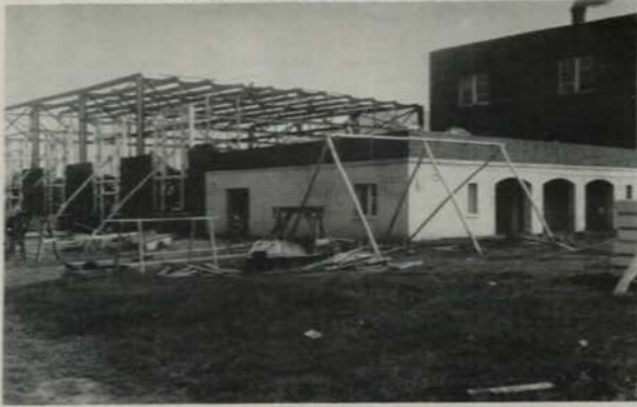
This view shows the construction of the school auditorium and additional rooms in 1928. Expansion of Joe Bradley School was undertaken several times by Merrimack Mfg Co., after they built the first section in 1919. (Photograph Property of Huntsville Parkers)
