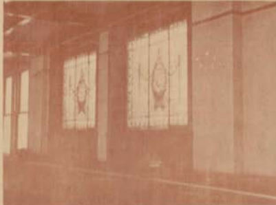
Interior, Balcony above Waiting Room, Union Station
