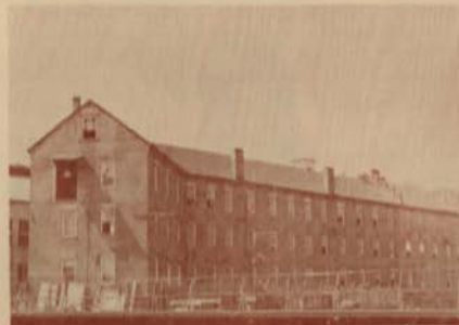
Creekside Building, Pratt Gin Factory
