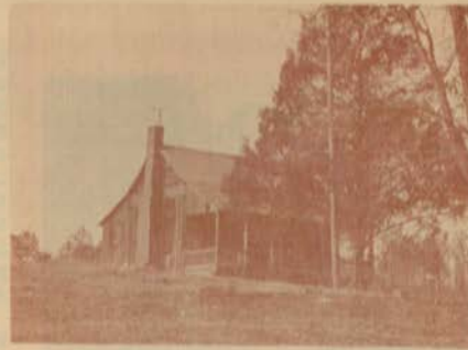
Rustic Cabin, Rural Elmore County
