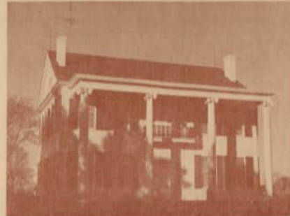
South Facade, Montgomery-Whittaker Home, Prattville
