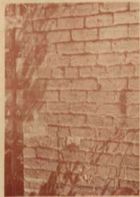
Detail of Brick, Back Building
