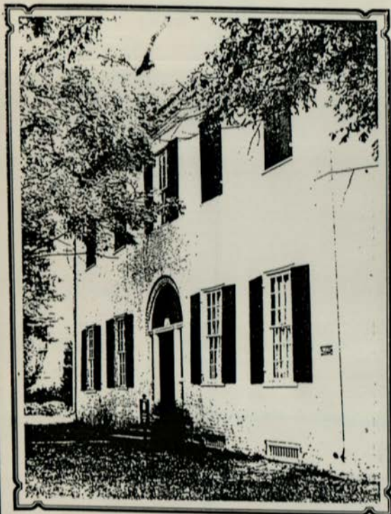
WEEDEN House, 300 Gates Street; entry featured on COVER.
