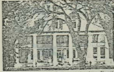
Figure 3. Southern mansions typify climate conscious design. The wide roof overhangs, exterior porches, shade trees, heavy masonry walls (painted white), and living quarters on the second floor (in each evening breezes and escape the radiant heat from the earth's surface) all are energy saving characteristics which provide reasonably comfortable living spaces without mechanical air conditioning. (Photo: Marcus Aumann Smith)
