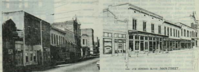
Figure 1. Inappropriate storefront alterations over the years—metal cladding, oversized signs and canopies—have detracted from the character of this historic district in Van Buren, Arkansas. A carefully considered rehabilitation plan for Main Street, including the removal of poorly designed signs, false fronts and the selection of an appropriate exterior paint color palette, serves to enhance the visual environment and preserves the district's sense of time and place. Photo above: Bob Dunn; Drawing, David Fitts
