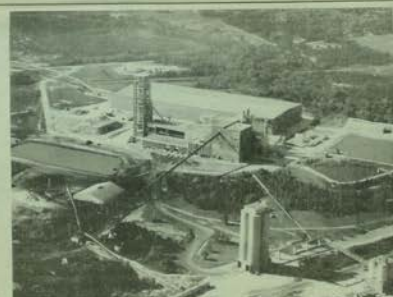
The plant began at the turn of the century, established by a British company. The company has merged several times: Lone Star to Citadel to General Portland to Lafarge. They built on and use massive amounts of Selma clink, which is a major ingredient in their products. The very thing that brought ruin to the Vine and Olive Colony is now utilized and very important to our industry.
