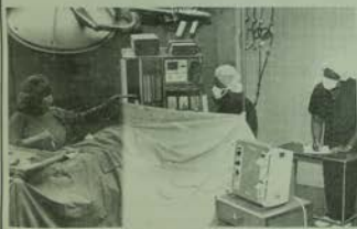
Operating Room, BWWMH in Demopolis Circa 1938
