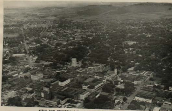
AERIAL VIEW, DOWNTOWN DISTRICT OF COUNTY SEAT, HUNTSVILLE, 1930
