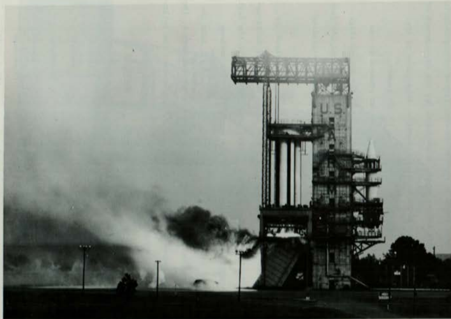
STATIC FIRING OF SATURN BOOSTER
