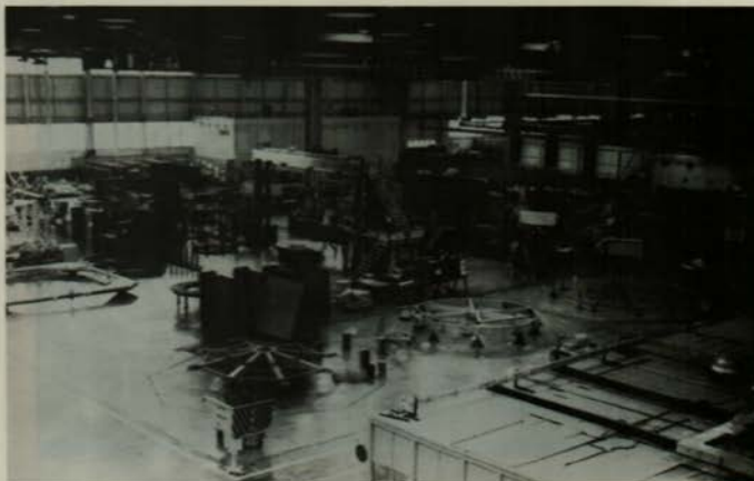
FIGURE 206. CHRYSLER SATURN IB FABRICATION AND ASSEMBLY AREA AT MICHLOUD
