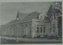
The Fort Payne Depot is an excellent example of Richardsonian Romanesque architecture.
