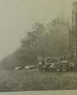
Drilling of new well #7-103 by a rotary drilling rig.
