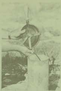
Ground-water quality varies with the elevation of the water table in the landfill area increasing the importance of water-level measurements.
