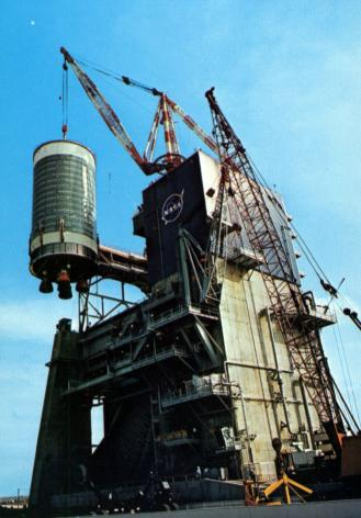
A ground test model of the Saturn V second stage (S-11) is lifted into a recently completed captive test stand at the Mississippi Test Operations in Hancock County, Miss. The NASA-Marshall Space Flight Center's Mississippi Test Operations will be used for captive firing the S-11 flight stages. Ground test stage was manufactured to test out S-11 systems and the ground test facilities.
