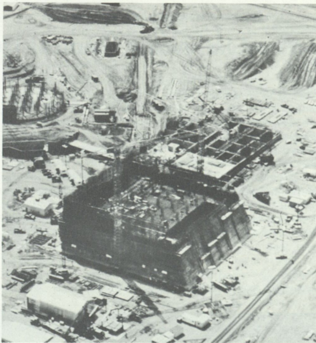
THE PERIMETER ACQUISITION RADAR (PAR), the long range eye of the SAFEGUARD Ballistic Missile Defense System, being constructed near Grand Forks, North Dakota, as it appeared in late July 1971. The PAR control building is front center, the 15,000 kw power plant directly behind, and the almost 4 million gallon capacity heat sink on top left. The facilities are being built under the supervision of the Grand Forks Area Engineer, Huntsville Division, US Army Corps of Engineers.
